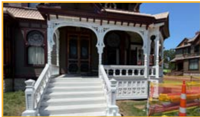
Repairs to the Hackley House
