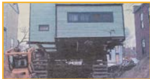
Repairing the foundation of the Scolnik House of the Depression Era
