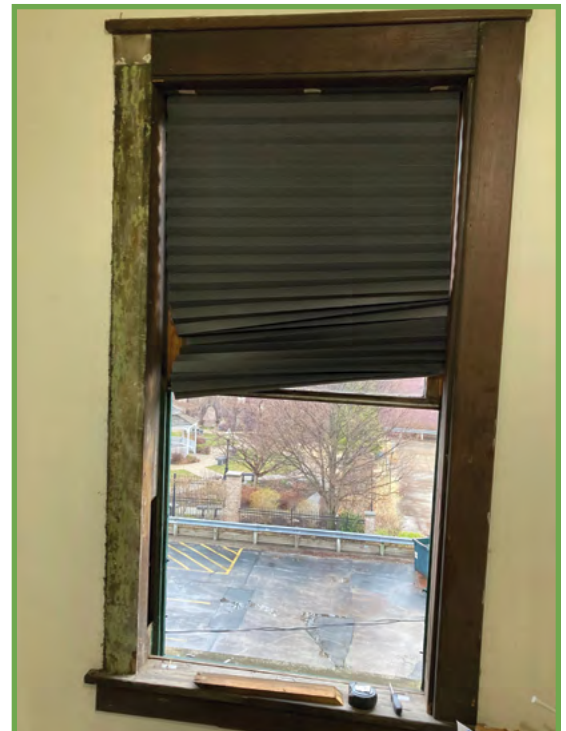
The right hand side of the window has its interior trim. The left side shows the inside face of the weight pocket box. The open gap on the left is the access door for the sash counter weights.
