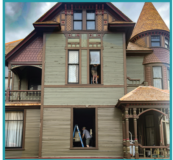
Windows are removed from the Hume House and taken to Grand Rapids for restoration.
