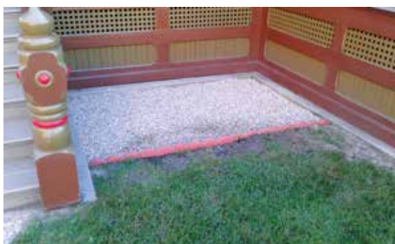
Soggy area at Hume Home resulting from roof runoff
